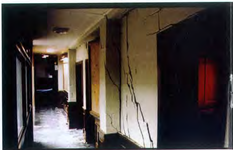
Figure 4. Building damage due to loess collapse.
